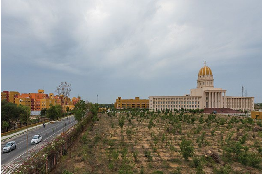
PICTURE 3: Pantation after construction
