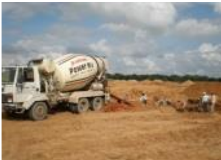
PICTURE 2: Construction of MUJ
