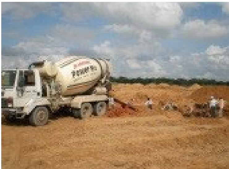
PICTURE 2: Construction of MUJ
