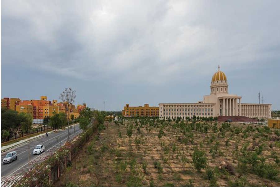
PICTURE 3: Pantation after construction
